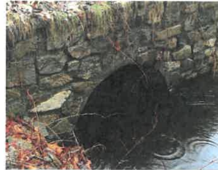
Figure 2 Existing pipe under Cobb Road
