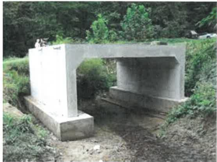
Figure 11 A unit like this can also be used, prefabricated/ prestressed concrete. We looked at this as an option.
